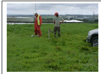
Load cell on truck winch
