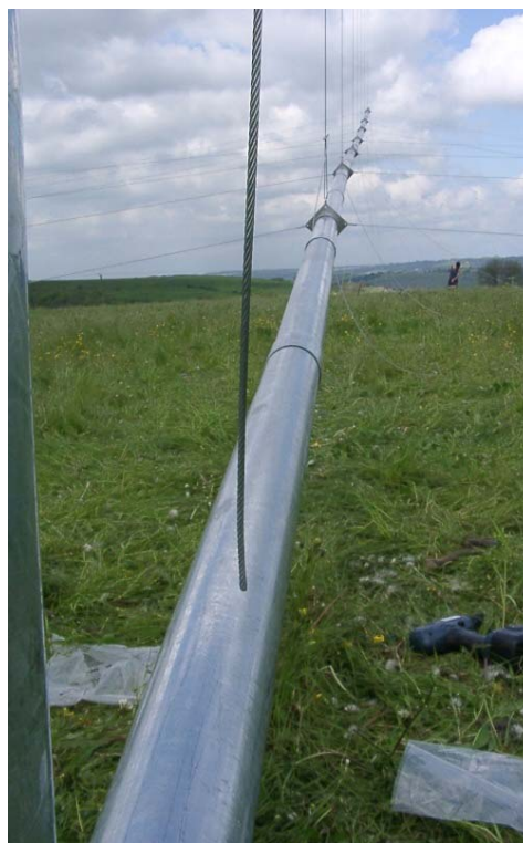
Snaking minimised during lift
