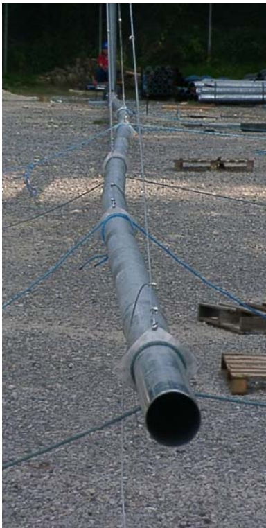
Snaking with insufficient side guy tension at initial lift
